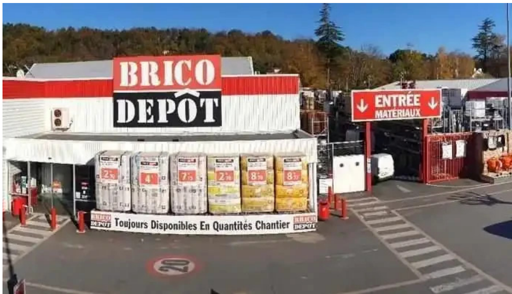
Brico depot photos du proprietaire
